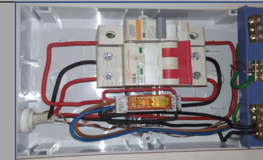
Relay Circuit / Manual Switch
